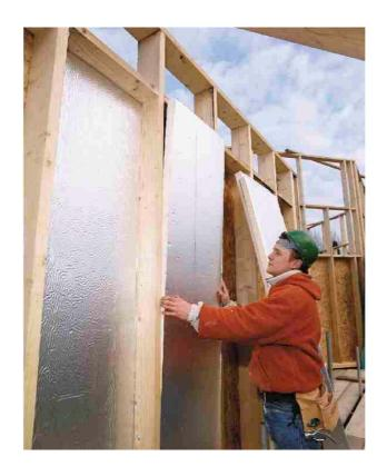
Kingspan Insulation's Kooltherm K12 Framing Board has passed a strict fire test, when tested to BS 476 Part 21.
